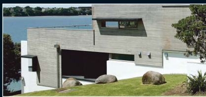
Stanley Point House
