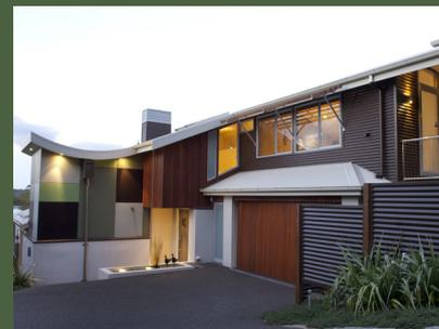
The roof has been purposefully picked out in a light colour for two reasons. From the lake, the roof is barely visible, therefore not a dominating feature. Approached from above the roof is read against the lake which is mostly reflective of the sky and clouds, thus a light coloured roof was chosen.
