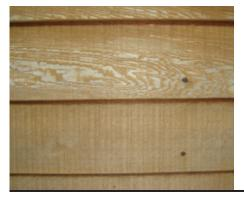
into parts of flat sawn weatherboards and tend to weather more rapidly (and require restaining sooner). The upper board in the photo below is flat sawn and has weathered much more than the quarter sawn board beneath it.
