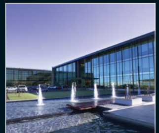
IAG Centre Wilson & Hill Architects Ltd
