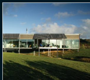
Kaitawa Rd House Dave Launder Architect
