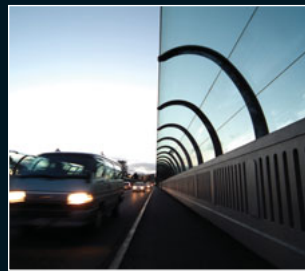
Grafton Bridge Safety Screens GHD Limited
