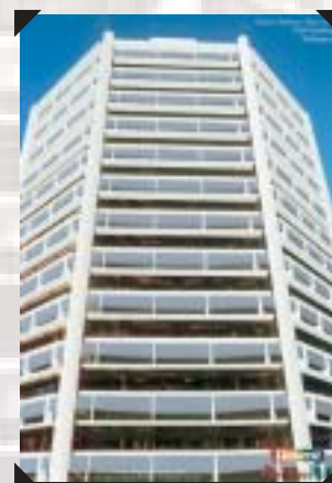
Confirming the colour scheme with RenderRite - this is what the finished project should look like.
