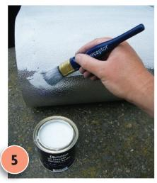
Apply one coat of Resene Waterborne Smooth Surface Sealer to the aluminium roof. Leave for two hours to dry.
