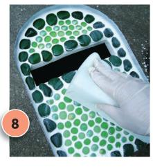
Mix the grout, according to instructions. Wearing latex gloves, work it into the gaps between the pebbles and nuggets. Wipe off excess with a damp sponge. Once the grout has set, remove residue with a clean cloth.
