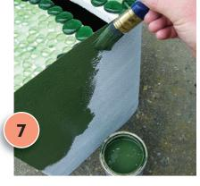
Paint the roof, back panel and 'door' with two coats of Resene Palm Leaf. Allow two hours for each coat to dry. Fix the door in position with the stainless hinges and screw the latch in place.
