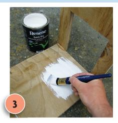
Apply a coat of Resene Quick Dry primer to both plywood mailbox sides. Allow to dry for two hours. Paint the mailbox inside with two coats of Resene Nero. Allow two hours for each coat to dry.
