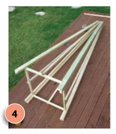
Attach the four 1.74m lengths of timber halfway between each corner support to form central upright supports, fixing at the top and bottom with 30mm screws and PVA glue – again, be sure to drill pilot holes first.
