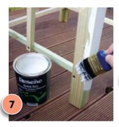
Leave overnight for glue to dry. Then fill any slight gaps between the obelisk and the finial with exterior filler. When the filler is dry, apply one coat of Resene Quick Dry to the entire structure, allowing two hours for it to dry.
