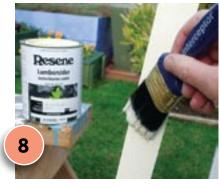
Apply two coats of Resene Colonial White to the entire structure, allowing two hours for each coat to dry.
