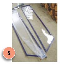
Nail two long lengths of the painted frame to each polycarbonate side panel with 20mm nails. Turn the panels over and attach two smaller lengths across the top and bottom in the same way. Fix at each corner with PVA and 40mm nails - drill pilot holes first to prevent the wood splitting. Saw off any excess wood. Remove the polycarbonate's protective film.
