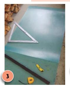
Measure and cut the polycarbonate sheet into the dimensions listed above, using a sharp craft knife to cut the polycarbonate.
