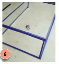
Cut four 1m lengths of painted framing and fix the side panels together, as shown, using PVA and 40mm galvanised nails - drill pilot holes first to prevent the wood from splitting. Use the set-square to ensure the frame is fixed at right angles.
