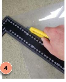
Make a mark on the front edge of both side panels 1450mm from the bottom edge. Draw a line from this mark to the back top corner. Cut along this diagonal line with the craft knife, as shown.
