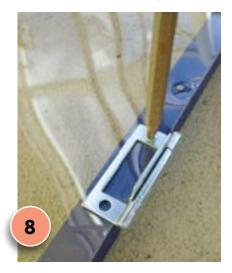
Attach the roof panel into position with 20mm galvanised nails and screw the door into position using zinc-plated hinges. Fix the hook and eye catch into position on the top of the door.
