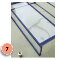
Measure the greenhouse front opening and make two panels to fit this space – one approximately 1400mm x 500mm (front fixed panel) and a slightly smaller approximately 1390mm x 500mm one (door). Spot prime and paint any bare wood where frames have been cut to fit. Fix the larger panel into position, as shown, using PVA glue and 40mm galvanised nails.
