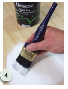
Fill screw holes and any imperfections and joints in the plywood with exterior filler. Sand smooth when dry. Apply one coat of Resene Quick Dry to all surfaces of the table and leave for an hour to dry.
