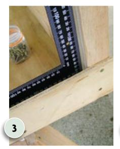
Ensure the first leg is at a right angle as you fix the plywood edging to the front support and table leg, using 40mm screws and PVA glue. Work around the table to fix the remaining plywood edging in the same way.
