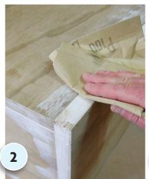
Fill any holes or imperfections in the plywood with exterior filler. Once dry, sand smooth with sandpaper.
