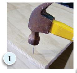
Using the plywood pieces cut as listed above, assemble the four sides of the planter using PVA and galvanised nails. Then position the base and fix it with PVA glue and galvanised nails. Drill drainage holes in the base.
