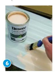
Apply two coats of Resene Manhattan to the smaller galvanised iron panel and allow two hours to dry between coats.
