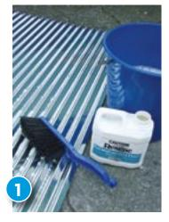
Mix up in the bucket one part Resene Roof Wash and Paint Cleaner with three parts clean water and apply to both sides of the galvanised corrugated iron and mini corrugated iron panels. Scrub vigorously with a hand brush and rinse off with clean water. Dry with a towel or old rag.
