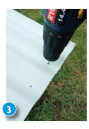
Attach the two lengths of 50mm x 50mm horizontally to the shed wall (approximately 1200mm apart) using 75mm stainless steel screws. Drill a series of holes along the top and bottom edges of the larger galvanised iron panel, as shown.
