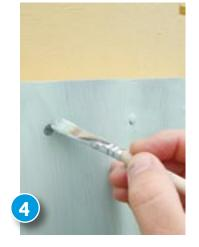
Attach the larger galvanised iron panel to the shed wall nailing 40mm galvanised flathead nails through the drilled holes and into the lengths of 50mm x 50mm timber. Use a small brush to spot prime the nail heads with Resene Galvo-Prime and allow to dry for four hours.
