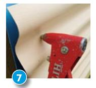
Position the smaller panel along the bottom of the larger panel and drill a 4mm hole through both layers of iron (making sure it's where two ridges touch). Fix into position with a pop riveter (following manufacturer's instructions), and repeat until the smaller panel is firmly attached.
