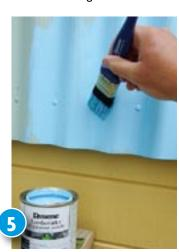
Apply two coats of Resene Malibu to the galvanised iron panel, allowing two hours for each coat to dry.
