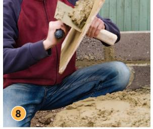
Mix a mortar of five parts sand to one of cement, enough to fill the cavities in the blocks. Fill them and hose lightly, ensuring the top of the second course of blocks has an even finish. Allow to go off. Once set, make a plaster (render) mix of three parts sand to one part cement. Add a dash of washing-up liquid as a plasticiser to make the mix smoother and easier to apply. Mix to a creamy consistency.
