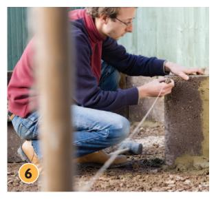
When it comes to making the curved edges of the bed, lay concrete blocks on their short ends (this is the exact height of the two blocks on top of each other used for the straight edges). This time, use a bed of mortar that is roughly 5cm deep. It's important to keep checking that the curved line matches up to the mark on the string tied to the pole.
