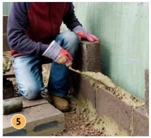
Lay the second course of concrete blocks on top of the first, using another bed of mortar, this time about 2cm deep. Make sure the two layers form a brickwork pattern, using a hammer and bolster chisel to cut blocks in half for the ends. Check the levels again.
