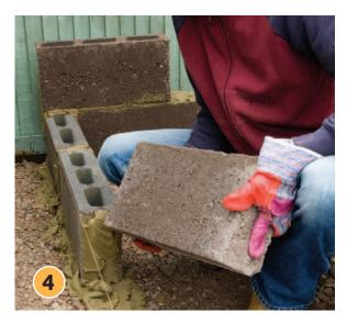
Mix a mortar of five parts builders' sand to one part cement. It's easiest to use a cement mixer, especially if you're building a large bed. Starting with the sprayed straight edges, lay the first course of blocks, placing them on their longest end, on a bed of mortar 5cm deep. Run a length of string between two pegs to help keep the blocks in a straight line. Use a spirit level to check the blocks are level.
