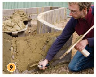
Apply the first coat of plaster to the blocks. It should be 5-10mm deep and it doesn't matter if it's quite crude. Cover the outside. You'll only need to plaster halfway down the inside of the bed, as the soil will cover the rest. Once you've finished, score large diamond patterns into the surface using the corner of your trowel. This is called a scratch coat. Wait for the scratch coat to go off overnight, then apply a second, smoother coat on top. Don't worry if the finish is a bit rough.
