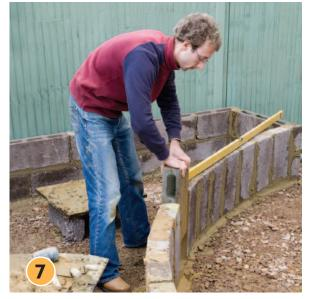
Lay the ends of the curved edges first, working in towards the centre. Carefully slot in the last block, cutting it to size if necessary. Make sure all edges of the bed are level on the vertical and horizontal, and tap them straight with a rubber mallet if necessary. Leave the whole thing to go off (set) overnight.
