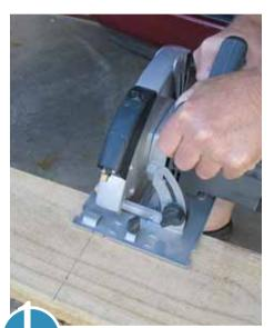
CUT timber to size. A circular or hand saw can be used, or ask your local building supplier to cut the wood to length. Sand edges with sandpaper.
