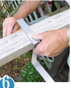
TO get an accurate measurement for the last bend, hold the steel pieces over the balcony rail and mark the bend with a pencil.
