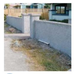
LEAVE freshly rough-cast concrete wall 28 days to fully cure before painting. Treat planting area with herbicide (or eradicate weeds by hand), remove any rocks or stones, lightly dig over and apply a 10mm layer of fresh top-soil.
