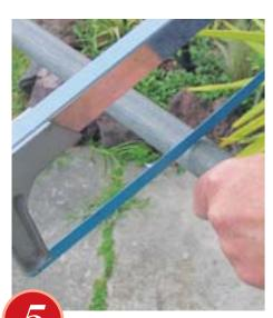
CUT two 50cm lengths from the galvanised pole using a hacksaw. These will be pushed into the ground to support the trellis.
