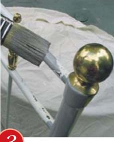
APPLY two coats of Resene Vinyl Etch to provide adhesion to the surface. If a clear lacquer covers the brass, remove this first with Resene Strip-Off.
