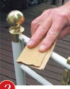
CLEAN the bedhead and lightly sand the enamel and brass surfaces. Brush away any remaining dust before painting.
