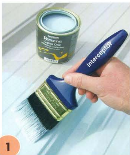
1 Prime both sides of the zincalume or colorsteel panel (if painting it) with a coat of Resene Galvo One (use Resene Galvo-Prime with brand new zincalume). Allow to dry for 12 hours. Clean out brush.
