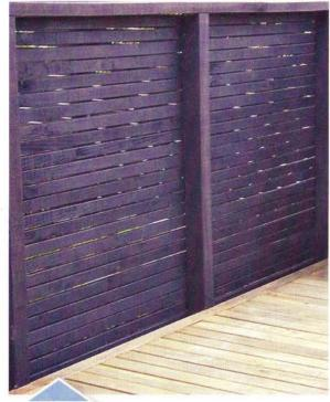
Give decking and wooden garden panels a makeover. First prepare the surface with a moss and mould killer. We used Resene Moss & Mould Killer and left it for 48 hours before washing it off with clean water. When the deck and fence were dry, we then used two coats of Resene Furniture and Decking Oil on the deck and two coats of Resene Woodman Penetrating oil stain in Resene Jacaranda on the fence.
