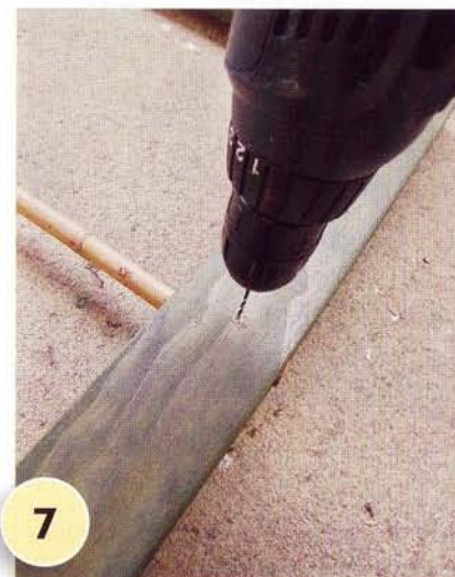
7 Slide a bamboo cane into position, aligning it with each mark. Drill a pilot hole through the frame's bottom edge and into the cane. Fix the cane with a 60mm nail.
