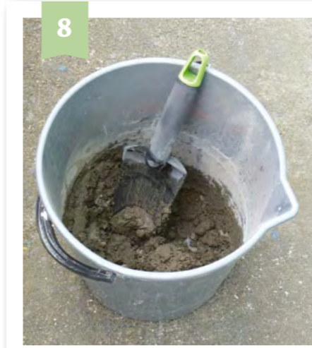
Mix a little builders mortar mix with clean water in a bucket to a fairly stiff consistency.
