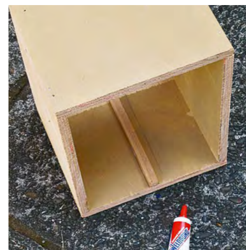
5. Measure, mark and cut two drawer runners from the 10mm x 10mm timber. Place one of the drawers inside the plywood unit and draw a pencil line along each side. Using this pencil line as a guide, fix the runners in place with PVA glue. Allow glue to dry.
