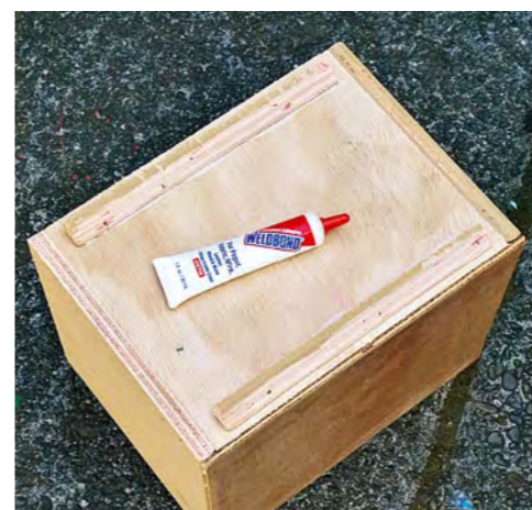
7. Measure, mark and cut two thin pieces of plywood (or offcuts of 10mm x 10mm timber) to form the base supports of the seed box. Fix these with PVA and allow glue to dry.
