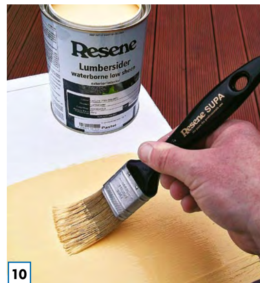
10 Apply two coats of Resene La Luna to the entire mailbox (inside and outside), allowing two hours for each coat to dry.
