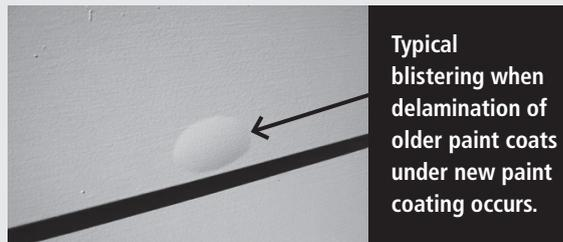
Typical blistering when delamination of older paint coats under new paint coating occurs.
