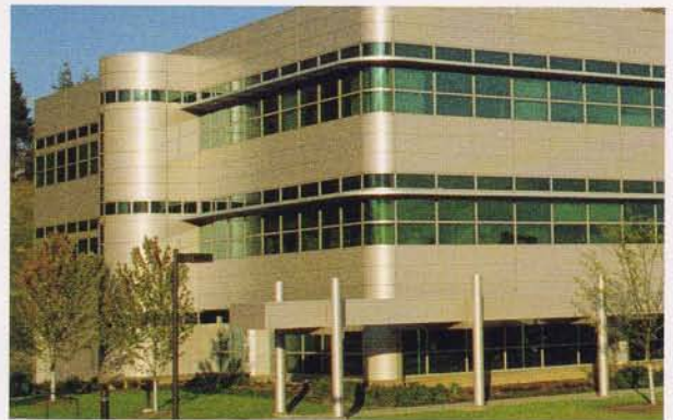
Colour on building exterior: Resene Metallic tinted to Gold Dust.
