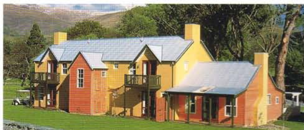
Timber walls: Resene Santa Fe
