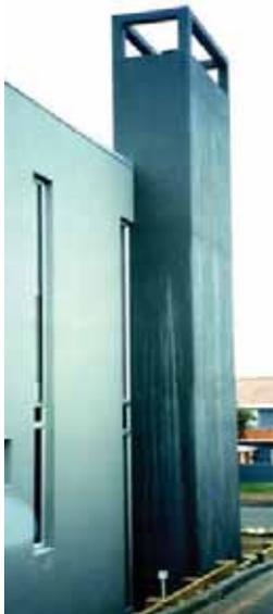
This results in loss of adhesion and/or it may 'burn' through the binder (resin) of ordinary latex paints, chemically altering certain pigments in the finished colour and weakening the film's integrity. In effect the paint will either flake off or be severely discoloured and this is most obvious with darker colours. The photo shows unsightly lime leaching through the painted plaster on this chimney.
