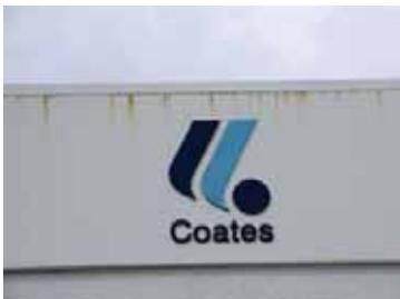
Providing the source of rust staining can be treated, seal the stained area with Resene Sureseal before overcoating with the selected topcoat system.
