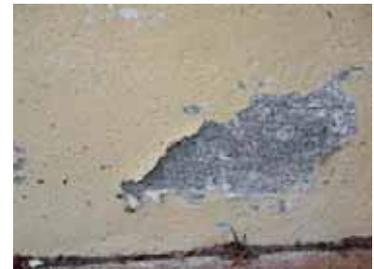
The alternative is to thoroughly scrub and wash to remove the worst flaking areas, spot prime with Resene Sureseal and paint with Resene AquaShield, Resene X-200 or Resene Lumbersider.
