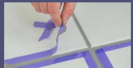
4: Carefully mask around the grout and paint on Resene Walk-on in your grout colour.
