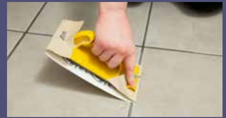
1: Lightly sand and clean the tiles and grout.
