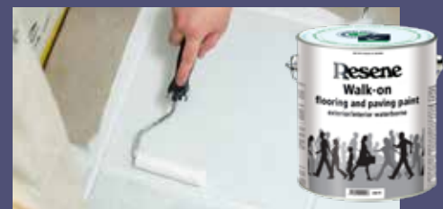
3: Apply two coats of Resene Walk-on to the tiles and grout.
