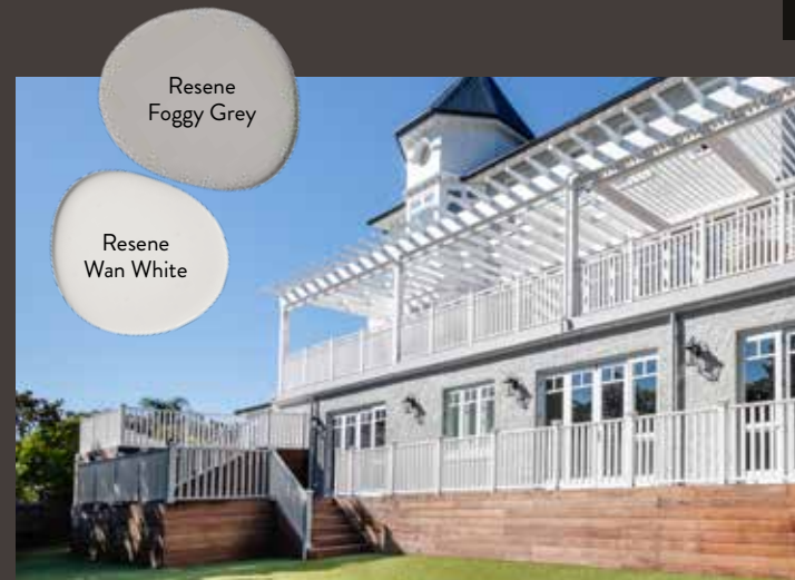
above: John's Arney Road Residence project won a Resene Total Colour Neutral Colour Maestro Award and features Resene Foggy Grey and Resene Wan White. Design by Abri Architects. Build by Keith Hunter Builders, www.keithhunterbuilders.co.nz. Painting by PBF, www.pbf.co.nz. Image by Katrina Weidner, www.catchlights.co.nz.
