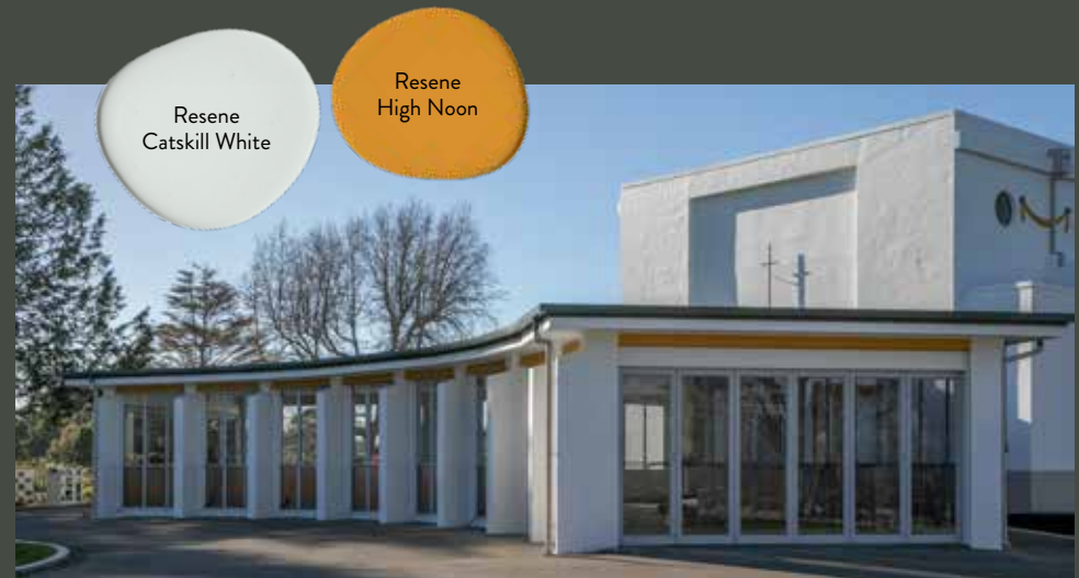
above: One of Susie's favourite projects to date was the Palmerston North Crematorium, which won a Resene Total Colour Heritage Colour Maestro Award and features Resene Catskill White, Resene Awaroa Bay, Resene Black Forest, Resene High Noon and Resene Greigewash. Design by Chapple Architecture. Build by Maycroft Construction, www.maycroft.co.nz. Painting by Martin Beveridge Ltd, www.martinbeveridge.co.nz. Image by Bernadette Peters Photography.
