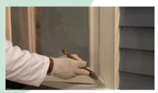
After completing the second sash using the same techniques and sequence paint the mullion rail.
