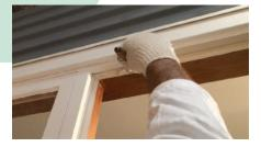
Start with the top edge and move down to the hinged side of the window jamb – painting both the inside face of the frame and the window before completing the opposite side and bottom inside face of the frame.
