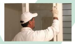
Next paint the top rail of the sash starting with the puttied edge - bringing the paint out over the putty and onto the glass by 1mm.
