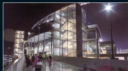
Jade Stadium West Stand Redevelopment
