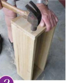
NAIL side, bottom and end pieces together to form two planter boxes. You can also use screws for greater strength.
