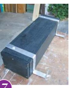
FIX steel pieces using bolts and washers (picture shows box upside down). Stagger the brackets to ensure the boxes fit back to back on the rail (see main picture).
