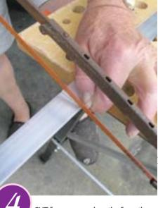
CUT four 500mm lengths from the steel bar using a hacksaw. File edges. Drill three holes in each length (see 7, which shows the bottom of the box, for spacing).
