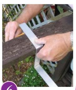
TO get an accurate measurement for the last bend, hold the steel pieces over the balcony rail and mark the bend with a pencil.
