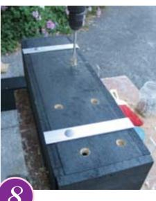
DRILL drainage holes, then line boxes with plastic, making holes in the plastic for drainage. For more on paints phone o800 RESENE or visit www.resene.co.nz
