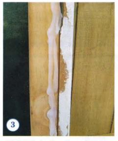
FOLLOWING the kitset instructions, erect the back and one of the side wall panels, running a line of silicon sealant along the join, as indicated. Fix with screws provided.
