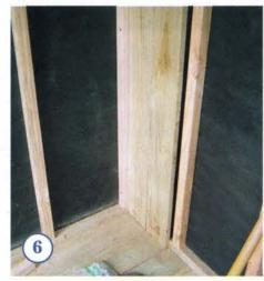
FINISH off roof interior and exterior trim following manufacturer's instructions, then line interior of the shed using fence palings. Attach top and bottom ends of each paling with two galvanised nails.
