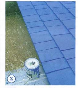
APPLY two coats of 'Resolution Blue' to the roof panels, allowing two hours to dry between coats. Lay the floor panel on a level concrete surface.
