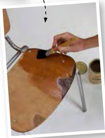
**TIP:** Don't use a solvent-based clear sealer unless you really need to. Resene Aquaclear Waterborne Urethane Varnish satin is an Environmental Choice-approved waterborne alternative. It's easy to apply and dries clear for a smooth, sealed surface
