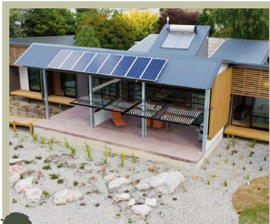
Above The house’s distinctive roofline gives it its ‘gullwing’ tag.
