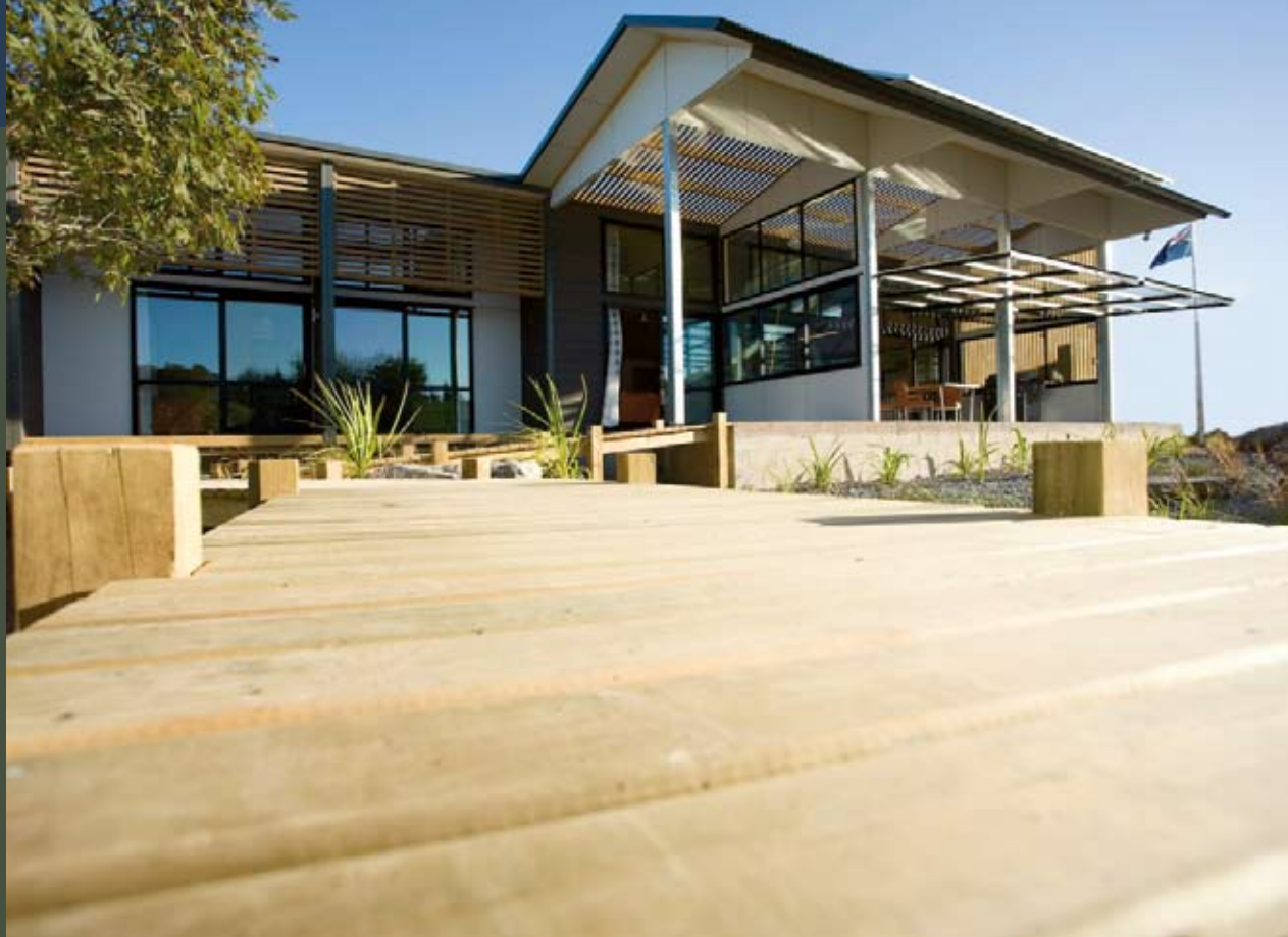
Right Large double-glazed windows on the northern side of the house welcome in the sun's warming rays.
