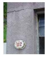
Hairline cracking often occurs as the cementitious surface (usually plaster or render) cures, especially if it is hot or dry, as water in the concrete mixture evaporates quicker than it would normally.
