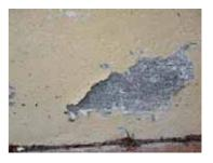
The alternative is to thoroughly scrub and wash to remove the worst flaking areas, spot prime with Resene Sureseal and paint with Resene AquaShield, Resene X-200 or Resene Lumbersider.
