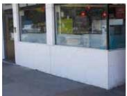
Compressed sheet is often used as a substrate for metallic finishes usually applied over a low to medium build texture, such as Resene Sandtex or Resene Thixalon 5.
