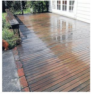
When the deck is dry, apply a coat of Resene Timber and Deck Wash or a similar product. This product cleans, but also enhances the stain penetration and assists in the longevity of the top coat.
