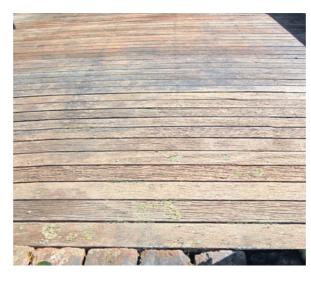
Clear the deck. ■ Use a sharp knife to remove as much of the moss as possible and to clear the spaces between the boards to encourage better drainage of surface water.
