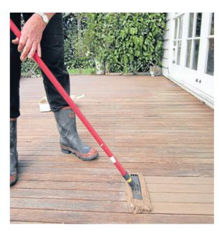
■ Ensure the deck is dry before you apply your stain with a long handle and a wonderful thing called a lambswool applicator – a fluffy cover that comes on a flat head that can screw on to a handle. Use a brush for the areas that are close to the house or difficult to access.
