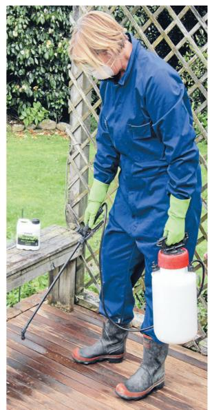
■ Put on your protective gear before spraying on a coat of moss and mould killer.
