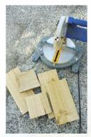
Measure, mark and cut the fence paling into the lengths listed above.
