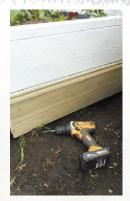
**Step 2**Fix into position using 90mm screws.
