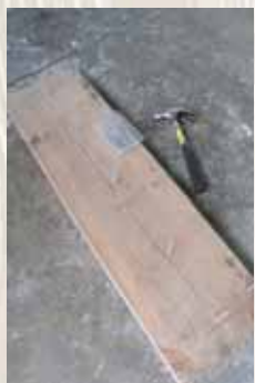
Step five Position eight nails along the seat, as shown.
