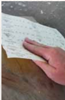
Step two Smooth any rough edges with sandpaper.
