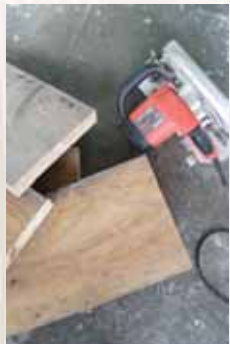
Step one Cut the timber to the dimensions as listed above.
