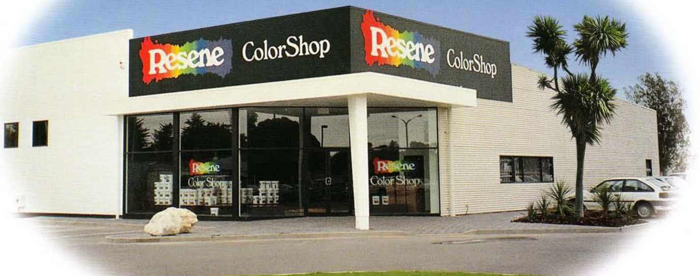
The new Resene ColorShop on Taradale Road in Napier.
