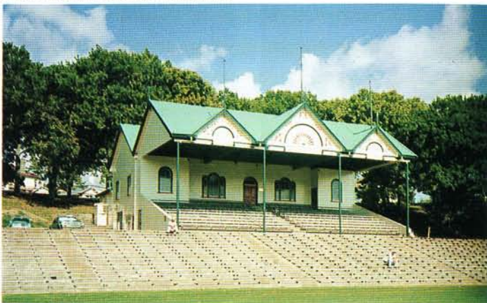
A famous Auckland landmark, the historic grandstand in the Domain was completely repainted by the Auckland City Council in preparation for the visit to New Zealand earlier this year of Pope John Paul II. Resene products were used entirely in the refurbishment of the grandstand. It was painted in Resene Super Gloss Enamel while Acrylic Hi-Glo was applied to the roof of the grandstand.
