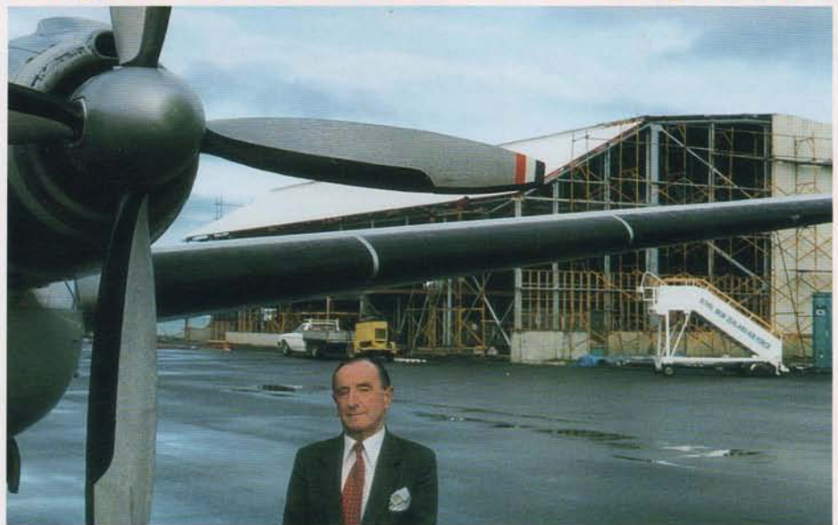
Resene Paints industrial coatings specialist Orton Moon in front of the new Ministry of Defence hangar at Wellington Airport that has been refurbished with the aid of Resene products. Steam and Sand of Petone did the sandblasting of the steel structure and the application of the new coatings.
