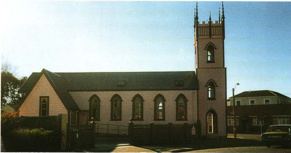
The refurbished St Mark's Anglican Church now the Headquarters of Norwell & Reilly, Architects and Consulting Engineers.
