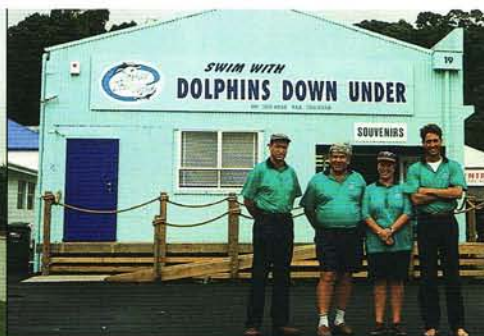
▲ Chambers on the town's river-front have been put to colourful use by tourism operator Dolphins Down Under . The company moved to its new premises, renovated with Resene paints, late last year. Pictured are co-principals Barry and Jo Wenham (centre) with staff members Doug Posa (left) and Craig Posa (right).
