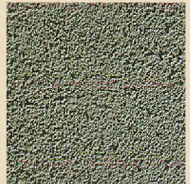
Scratch plaster finish
