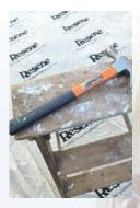
Step one Hammer in any protruding nailheads.
