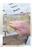
Step three Lightly sand any filled areas and wipe off any sanding dust with a clean cloth.
