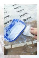
Step two Fill any overly large holes or cracks in the wood. Allow filler to dry.
