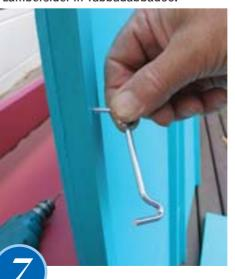
FIX two hooks to the supports on each end panel. Fix two eyes at corresponding levels to a wall or fence, for the hooks to latch into.
