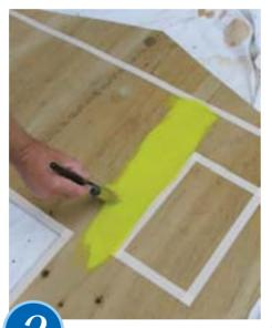
APPLY masking tape around the door, windows and roof to separate paint colours. Apply three coats of Resene Lumbersider in Neva (from the Resene KidzColour range).
