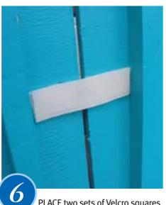
PLACE two sets of Velcro squares on one side of each panel, 200mm from the top and bottom. Attach longer strips of Velcro to join the two panels.
