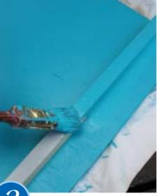
FIX supports to the insides of the four side panels, just in from the edges. On the two end panels, fix one of the supports on the very edge of the panel. Apply three coats of Resene Lumbersider in Yabbadabbadoo.
