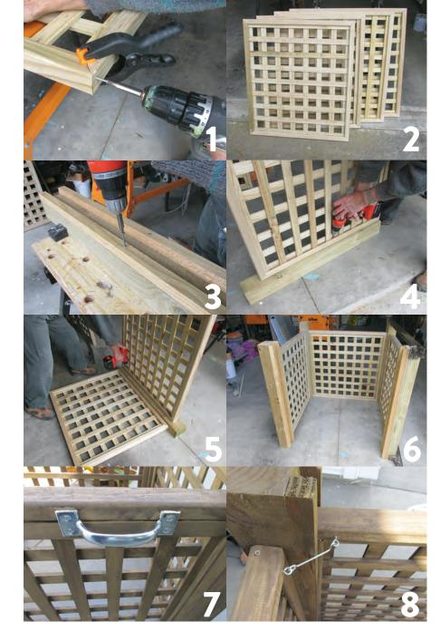
**1** Fit 4 x 720mm and 4 x 820mm capping lengths to the two smaller panels. Cut capping further, if necessary, to fit snug. Screw together, using 38mm screws.
