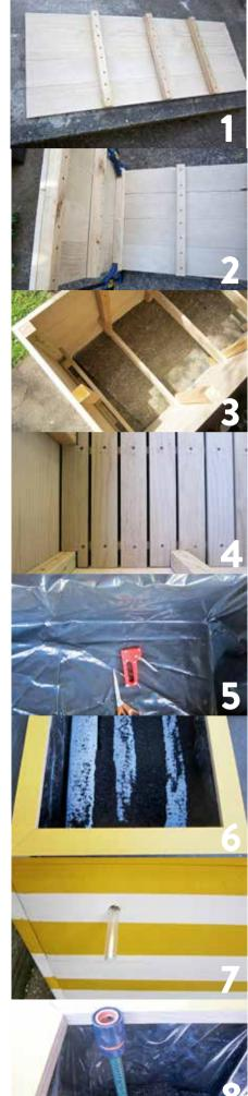
Lay four of the 600mm boards flat on the workbench and, keeping the assembly square, screw two of the posts at each end and one centrally, with two screws into each board. Repeat for the sides with two posts 340mm in from each end and one centrally.
