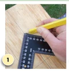
Measure pieces of plywood to fit the above dimensions. Use the set square's corner to mark the pitch of the gable roof on the front and back walls (the sides should each measure 250mm)
