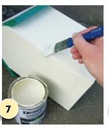
Nail and glue roof panel 1. to one side of the gable. Attach roof panel 2. to this with the hinge and screws. Paint the birdhouse exterior with two coats of Resene Colonial White.
