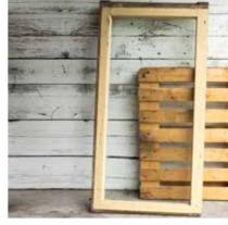
Step 1: Scrub the window sash clean with a cleaner and water. Coat exposed timber with Resene Quick Dry Primer Undercoat, and cover any existing old enamel paint with a coat of Resene Waterborne Smooth Surface Sealer. (You can do this instead of sanding the old paint.)
