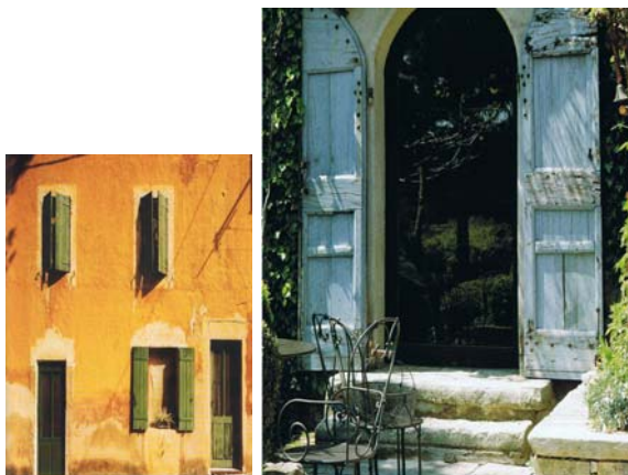
gates and shutters
